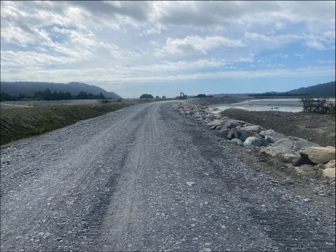
Looking up stream at the newly completed extension to the Milton & Others Stop bank
