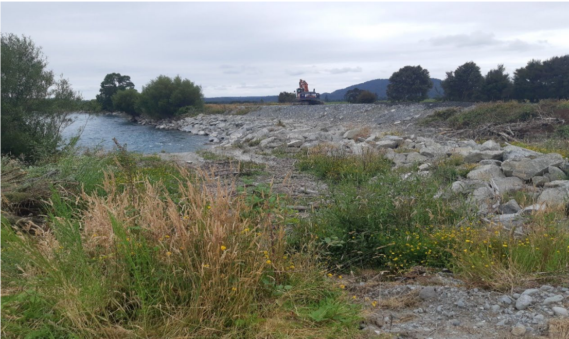
Site 3: A Henry Adams Operator repairing stop bank.
