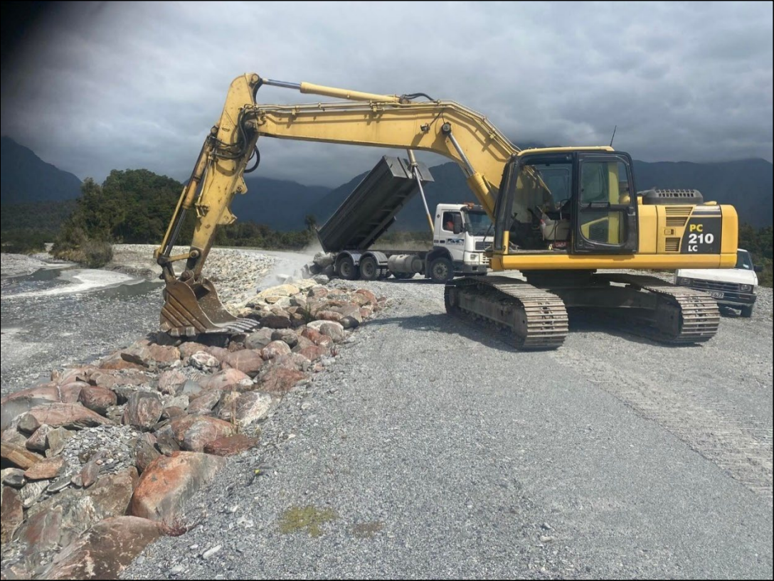
Looking up stream at the newly completed extension to the Milton & Others Stop bank
